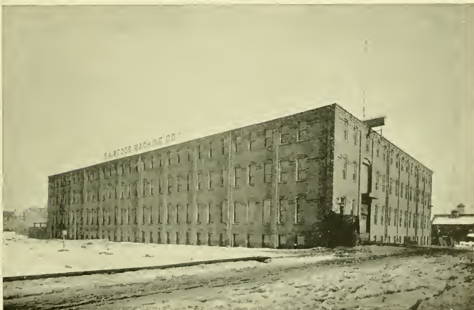
BUILDING OF THE S. A. WOODS MACHINE COMPANY.
